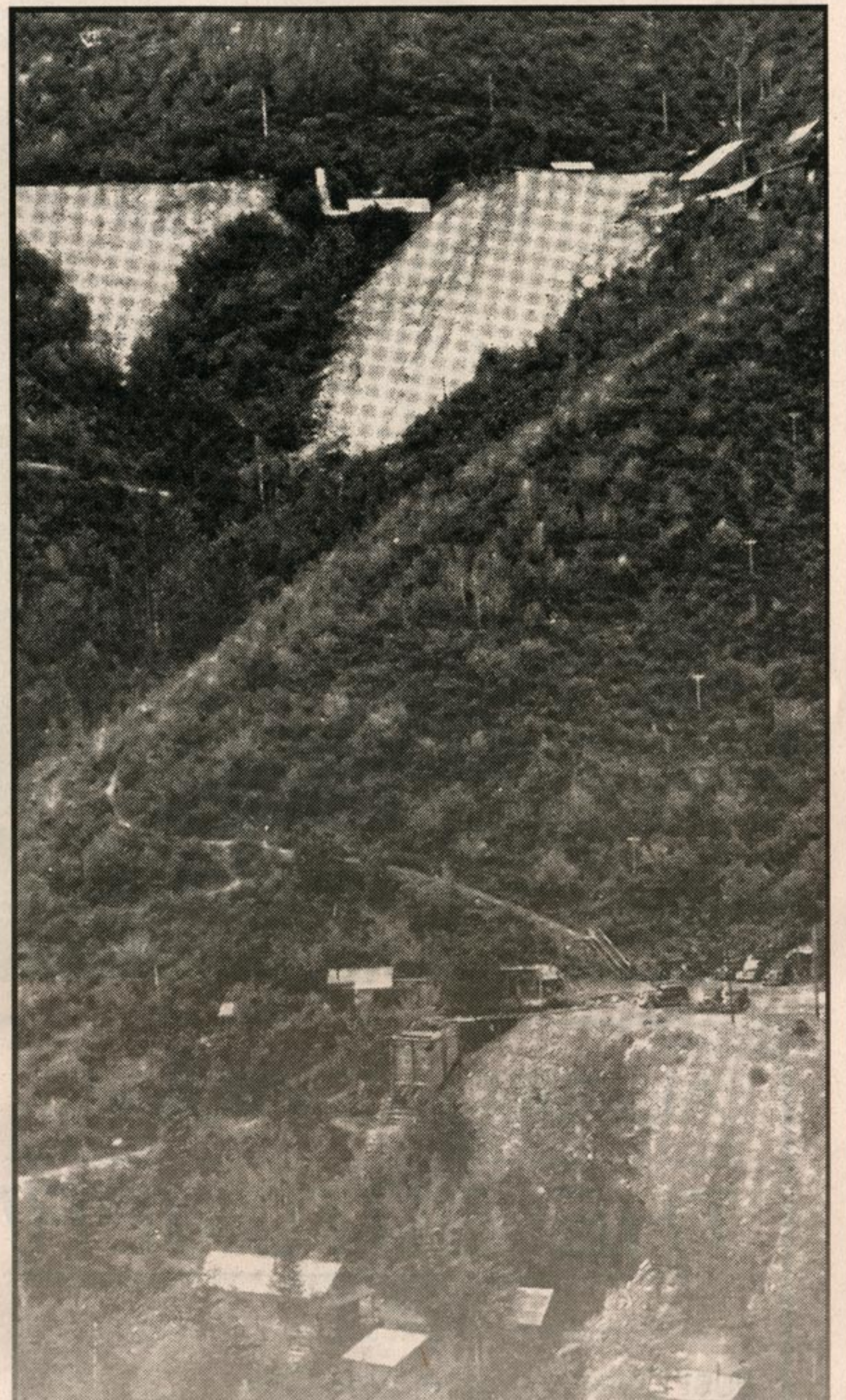
Mill Buildings at the Yankee Girl Mine 1934 Board of Trade photo 1934
